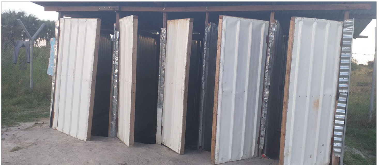
Pit latrines in Leer County Temporary Protection Area
